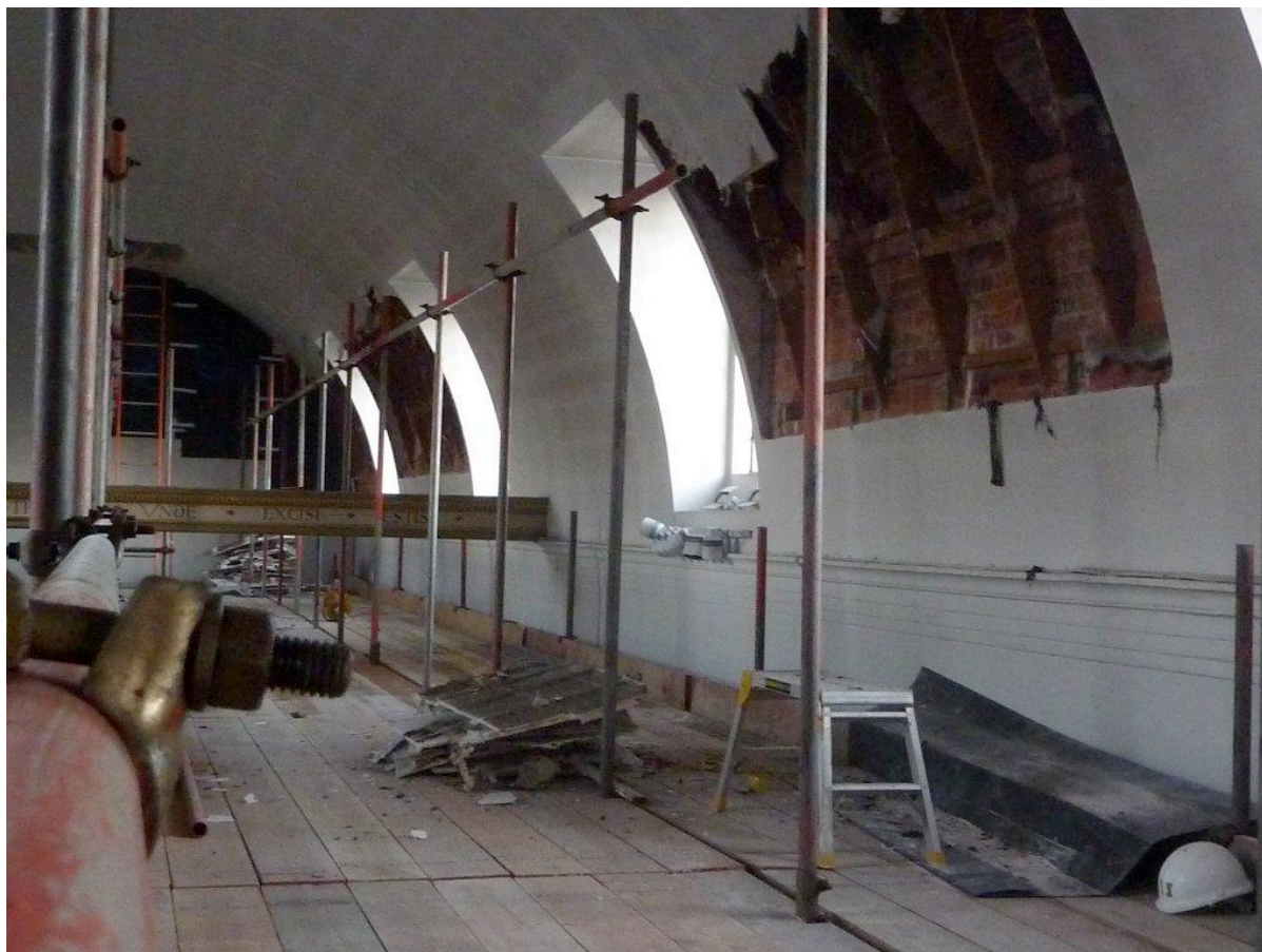
Photo showing partial removal of the south side of the ceiling.
