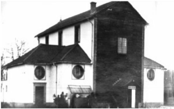
1. Partially completed church
